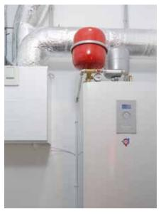
Thermia Diplomat Optimum 6 kW ground source heat pump
